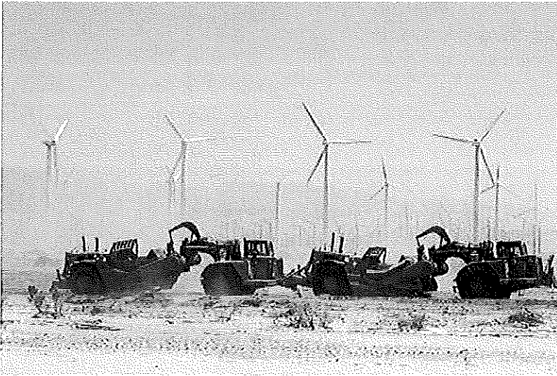
Large graders remove silt from the bottom of the percolation ponds in May so water can seep into the aquifer more efficiently. Jay Calderon, The Desert Sun
